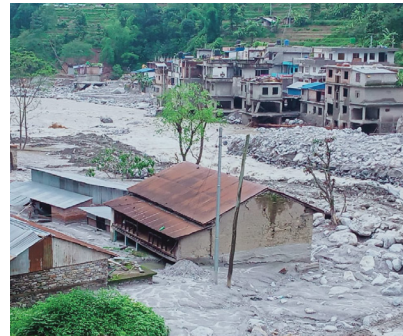
Destruction caused in Melamchi. – Photo by Arjun Shrestha
