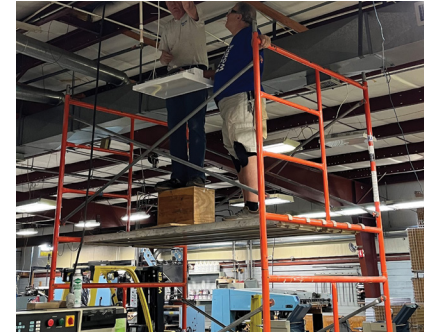
Volunteers Installing New LED Lighting in the Print Shop — Photo by Phil Winder
