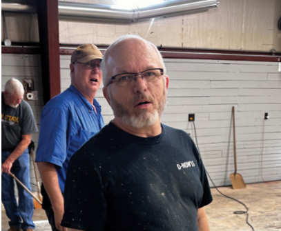
Phil As Part of the Crew on Concrete Work Needed for the New Press — Photo by Dan Winder
