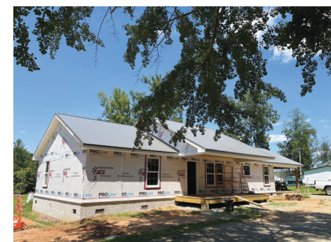
Current Construction of Campus House at SLM HQ — Photo by Phil Winder
