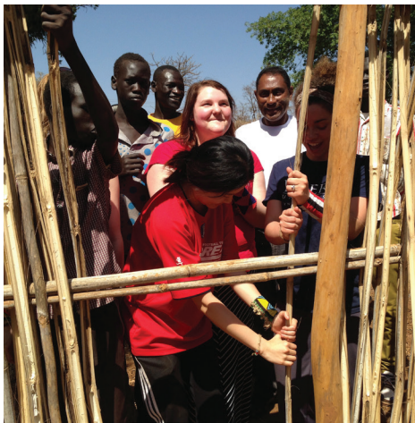
University Students Helping Rebuild the Church — Photo by Ron Barnes
